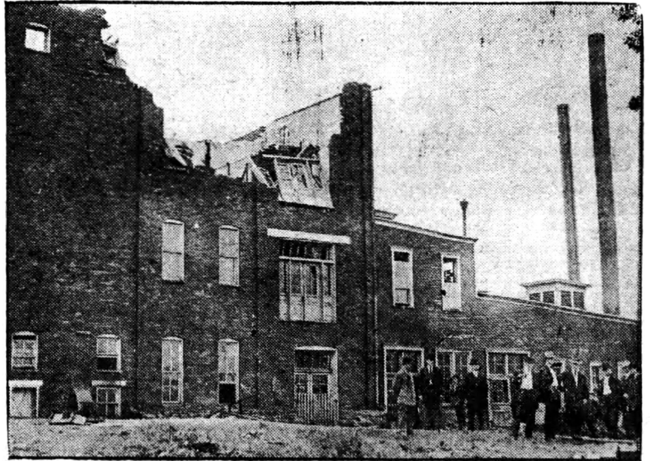
UNROOFED MEYERSDALE BREWERY.
